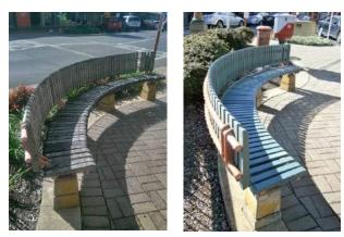
Replace or renew? Seats that have been a feature of Morrinsville's CBD for many years were given a complete makeover with frames re-galvanised and powder coated to look like new, plus recycled plastic slats machined to replicate the originals.
